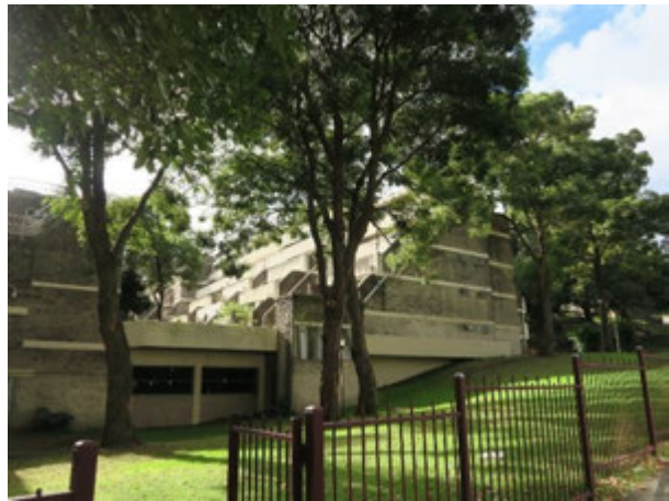
Picture 14 – Southern elevation of 'Dobell', taken from McEvoy Street
