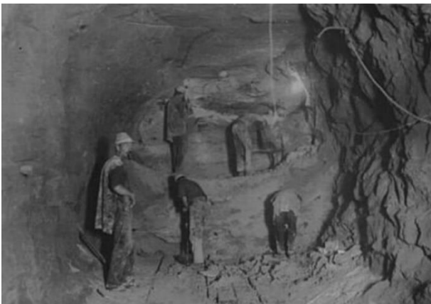
Picture 35 – Construction of the Pressure Tunnel between 1921 and 1935
