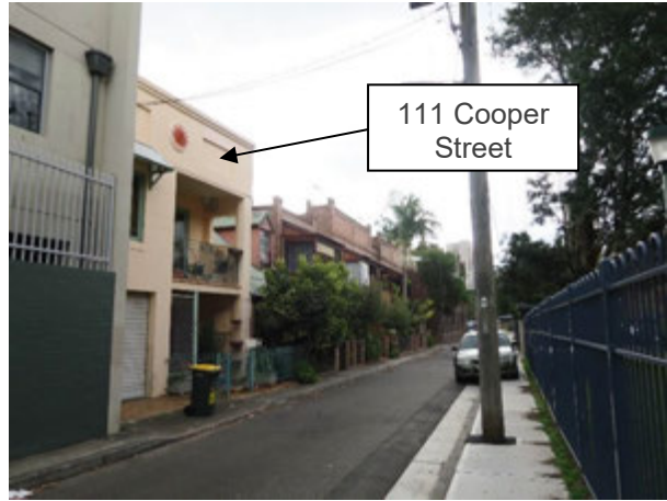
Picture 16 – Referential infill development at 111 Cooper Street
