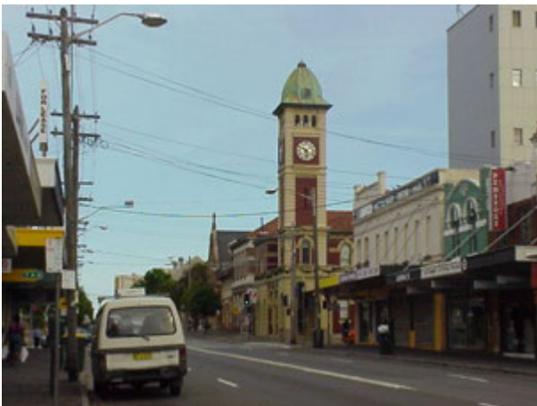
Picture 39 – View of Redfern Street.
