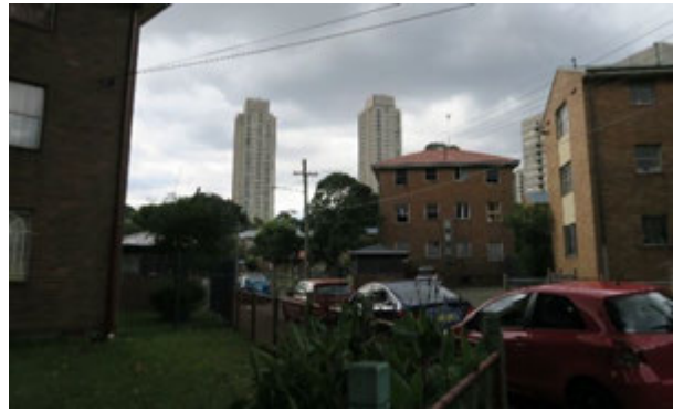
Picture 10 – Typical walk-up buildings facing north along Cooper Street, with Matavai and Turanga visible in the background
