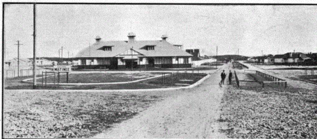
View down Cook Avenue, showing Picture Theatre and Social Hall.
