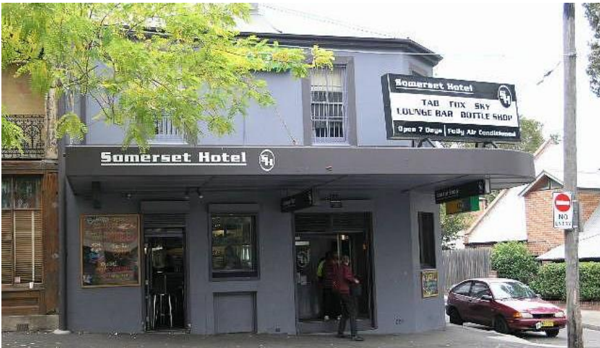
Figure 35 – Former Somerset Hotel, Pitt Street elevation.
