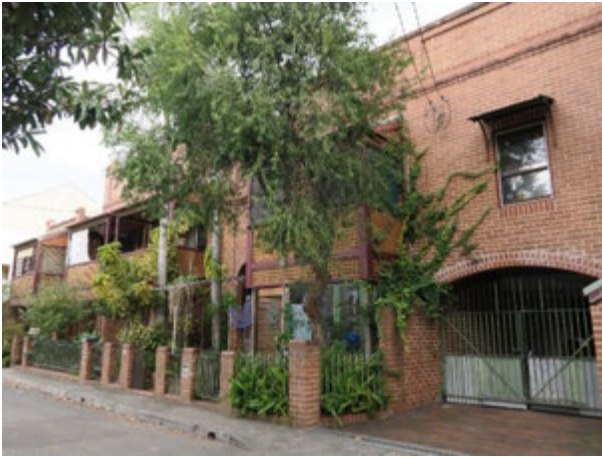
Picture 15 – Referential infill development at 97-109 Cooper Street
