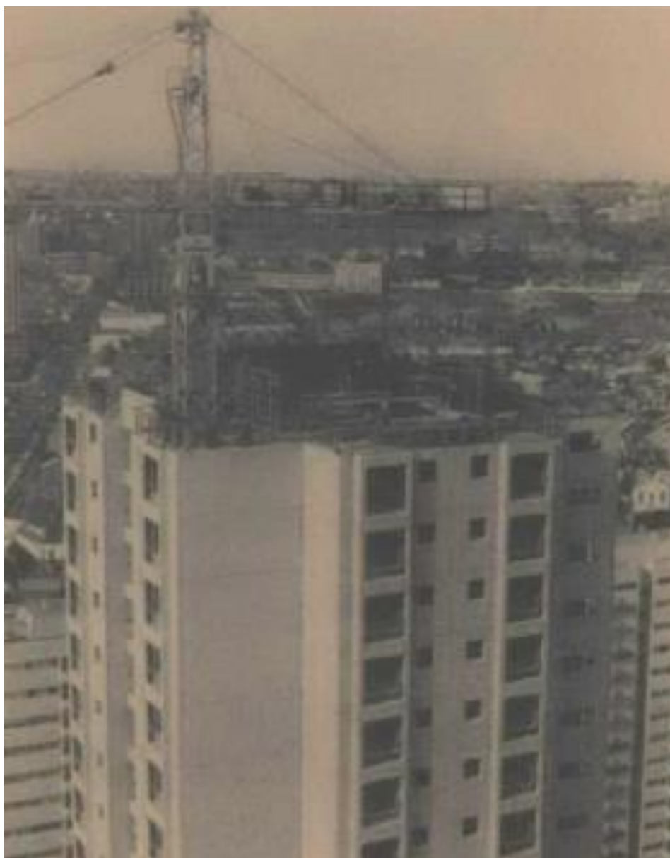
Figure 95 – View of one of the Waterloo towers during construction, c. 1975
