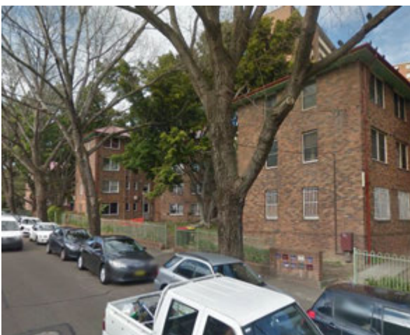
Picture 67 – Devonshire Street, Surry Hills (Google Streetview 2016)
