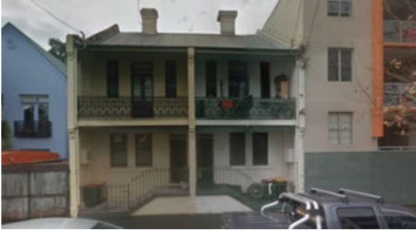
Figure 23 – View of terrace pair from Cope Street.
