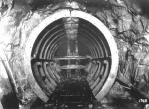
Picture 33 – Indicative view of the Pressure Tunnel
