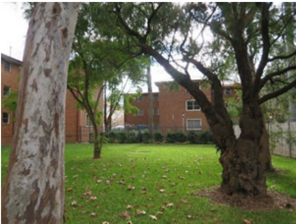
Picture 7 – Southern elevation of walk-up flats at 247-251 Cope Street, facing north from McEvoy Street
