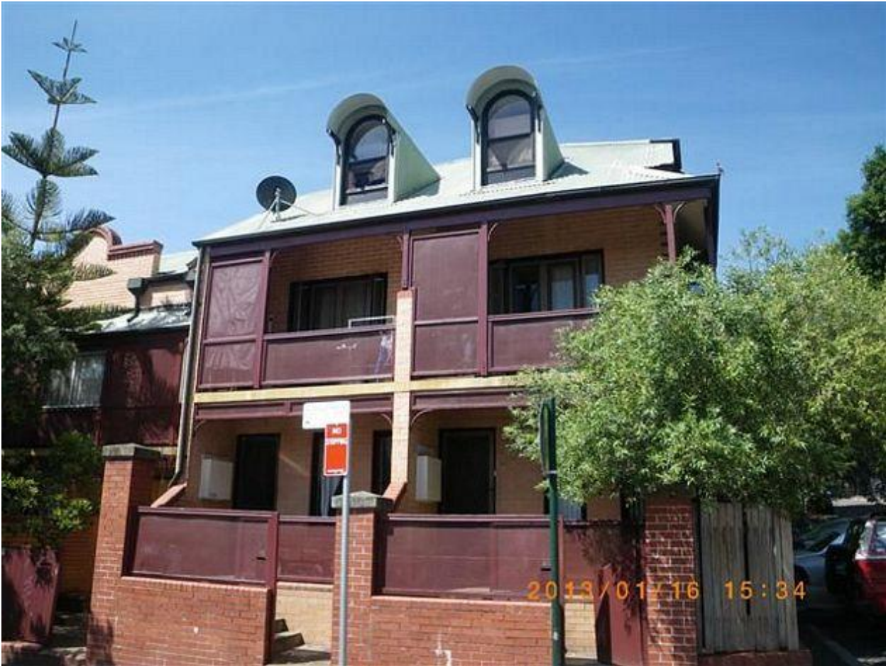
Figure 126 – View of the referential infill terraces at 82-96 Bridge Road, Pyrmont, dated 2013
