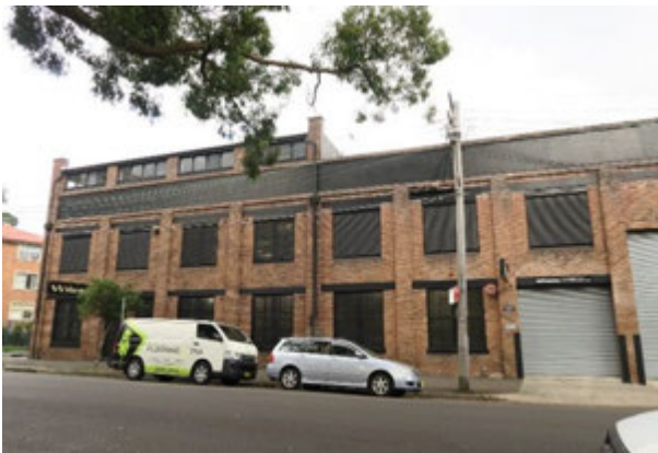
Picture 17 – Privately owned commercial warehouse building at 116 Wellington Street
