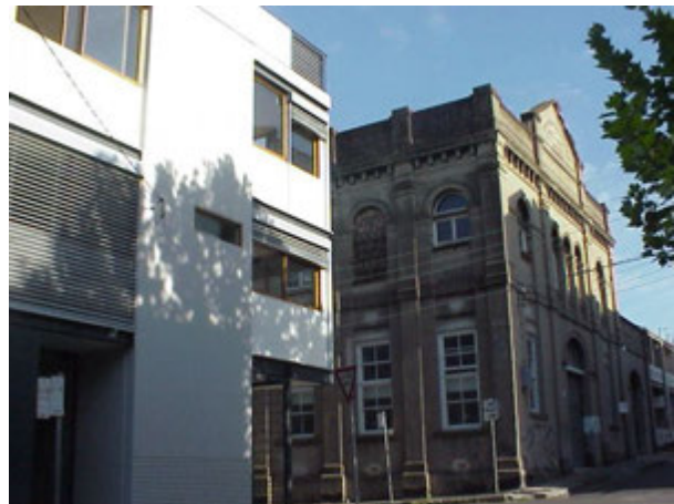
Picture 40 – View of Turner Street.
