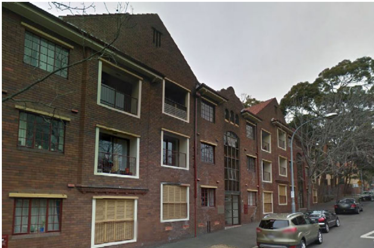
Figure 65 – View of the Dowling Street Flats
