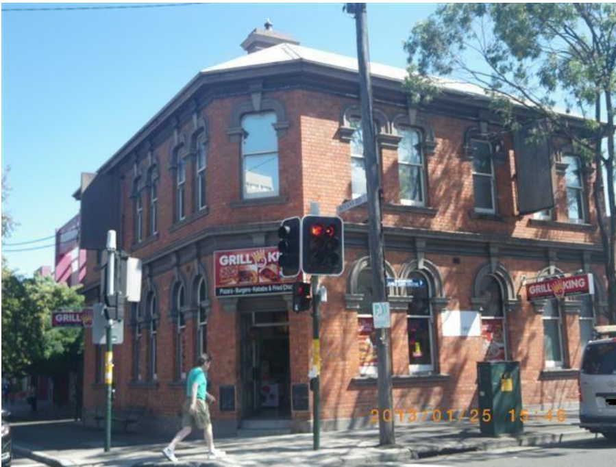
Figure 31 – Former CBC Bank, Henderson Road elevation.
