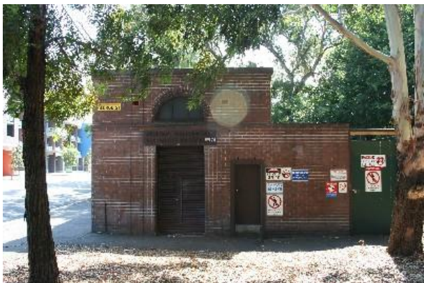
Figure 22 – View of Substation 174.
