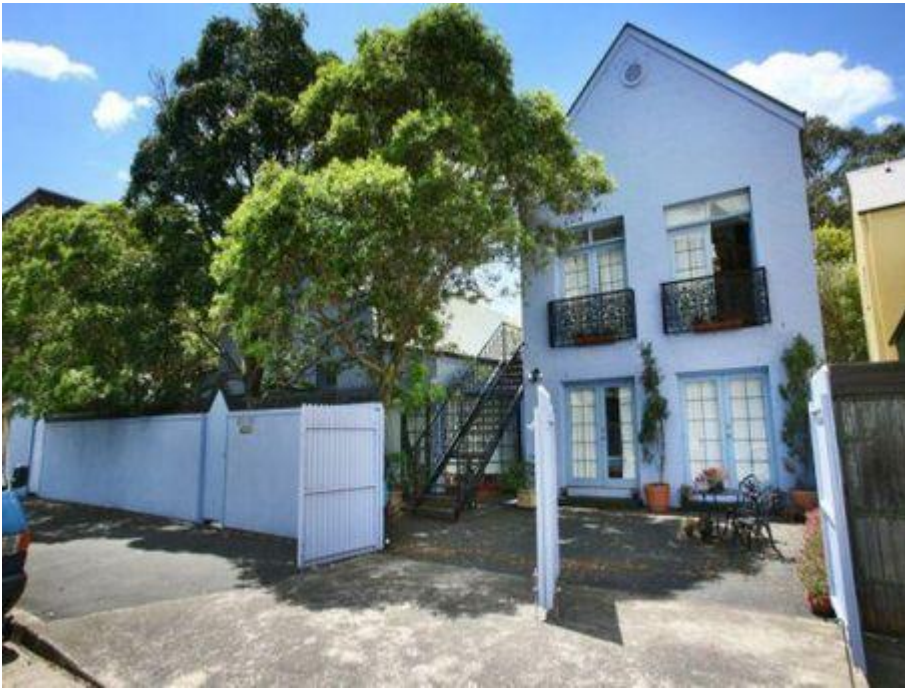
Figure 24 – Former Waterloo Pre-School as viewed from Cope Street.
