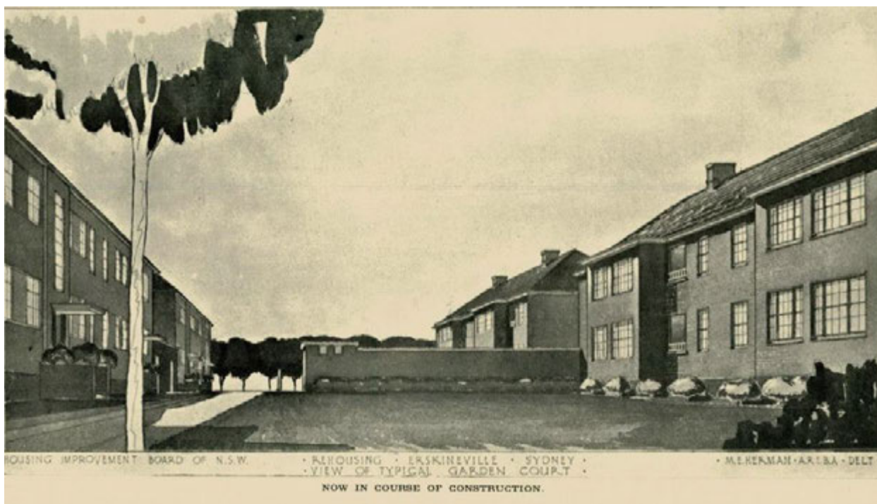
Figure 75 – View of the proposed Erskineville Estate during construction, c. 1938
