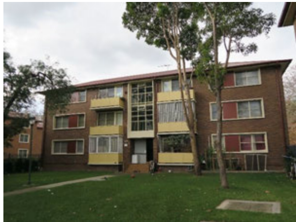
Picture 8 – 249 Cope Street, facing east
