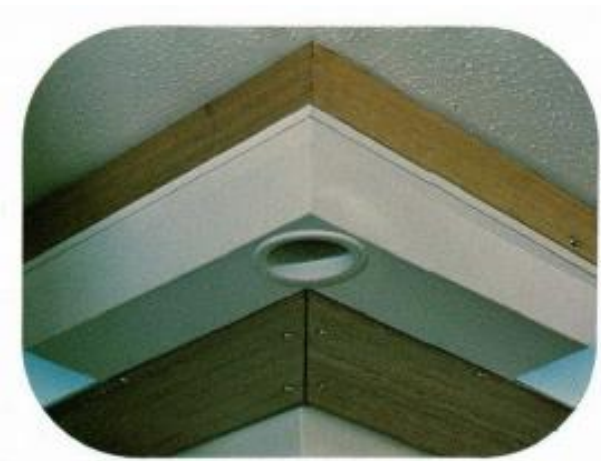
Picture 51 – A battery operated lighting system in the corridors and fire stairs, to ensure light is available in the case of power failure
