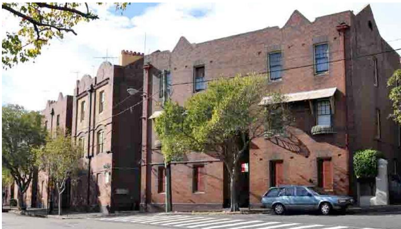
Figure 61 – View of the Lower Fort Street tenements, 2009
